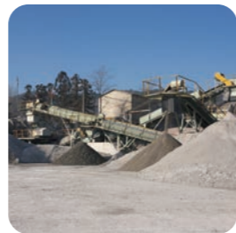
Debris processing facility
